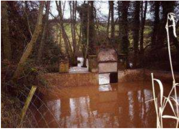
Above is the weir and sluice gate to hold back the stream to drive the water wheel for use by the mill.
