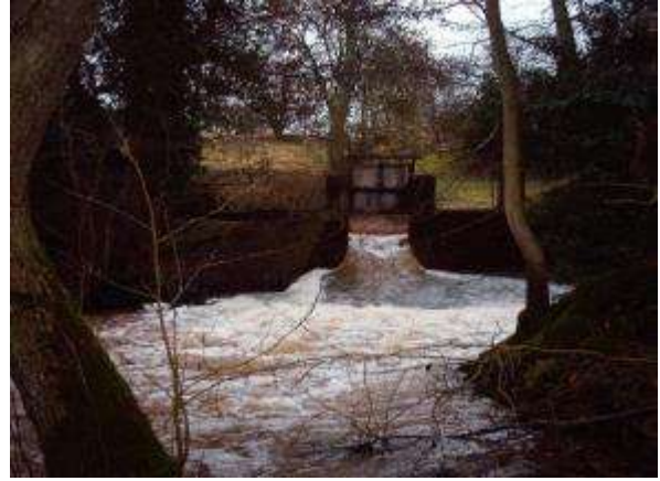
Above is the weir and sluice gate to hold back the stream to drive the water wheel for use by the mill.
