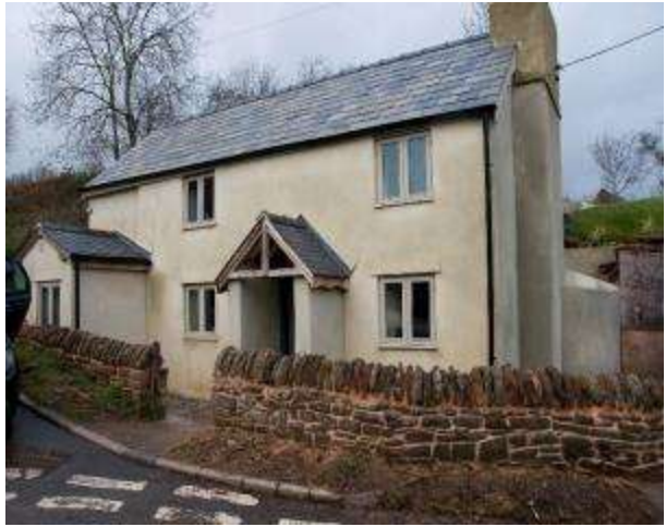
Across the junction from Rock Cottage is Cobblers Point - This was Stan's childhood home
